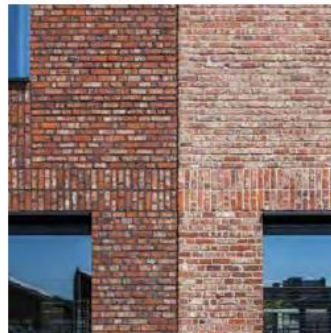
Double Stack Bonded Soldier Course/Brick Banding at First Floor Level
